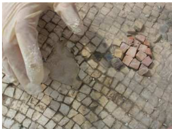
Fig. 9. One of the conservators preparing loose tesserae for replacement where the pavement was smashed by falling stones during the earthquake of AD 749 (photo: J. Burdajewicz)
