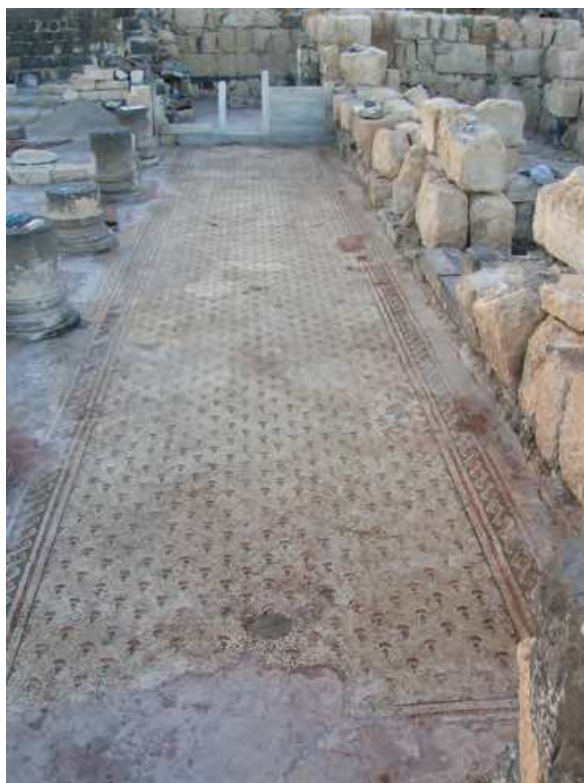
Fig. 10. The North-West Church needs a project for a proper exhibition of the mosaics in their architectural context. An overall plan of opening the site to the public should include a long-term conservation plan and the upgrading of some of the solutions applied during exploration. This will allow the mosaics to speak the site's history (photo: J. Burdajewicz)
