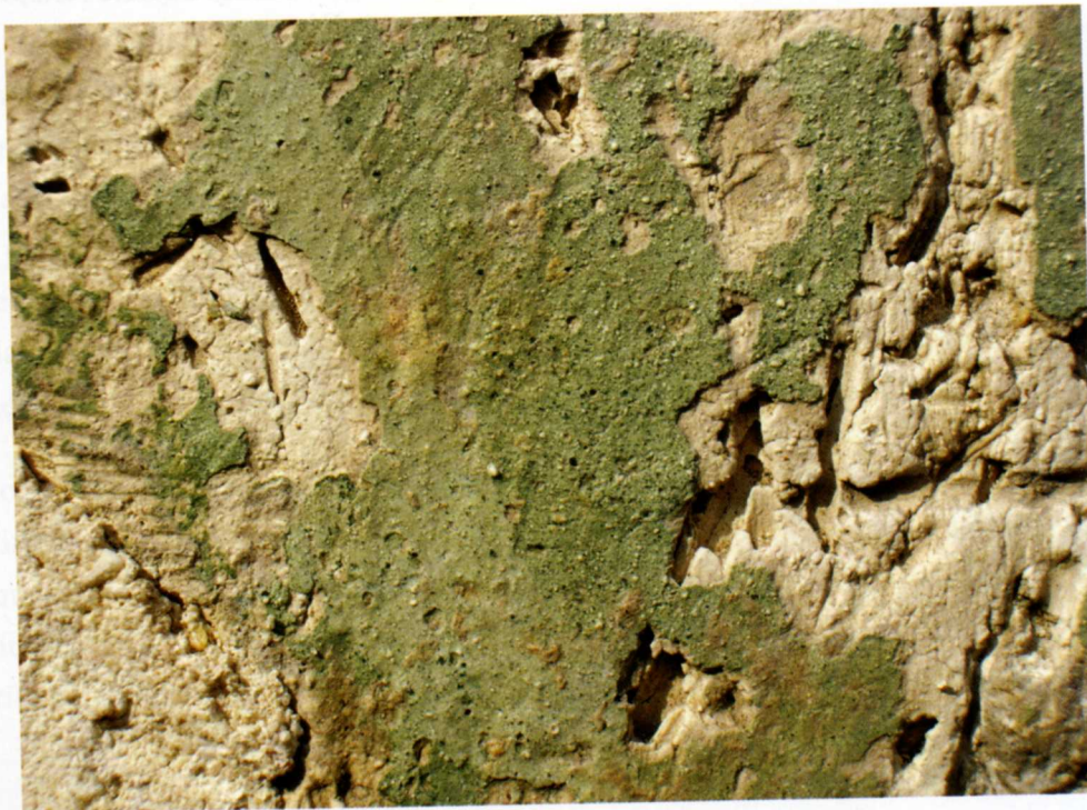
Fig. 3, Remains of green-coloured plaster covering columns' drums stored in the lapidarium by the northern entrance to the atrium . State of preservation after routine cleaning and removing of a thick layer of dirt (close-up).
