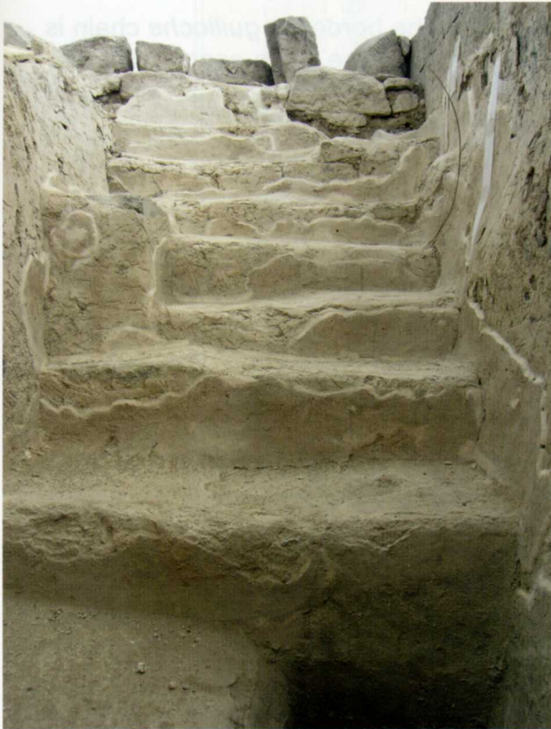
Fig. 81, Hippos, NWC, collection vat of the winery, steps descending to the pool. State after basic stabilization treatments.
